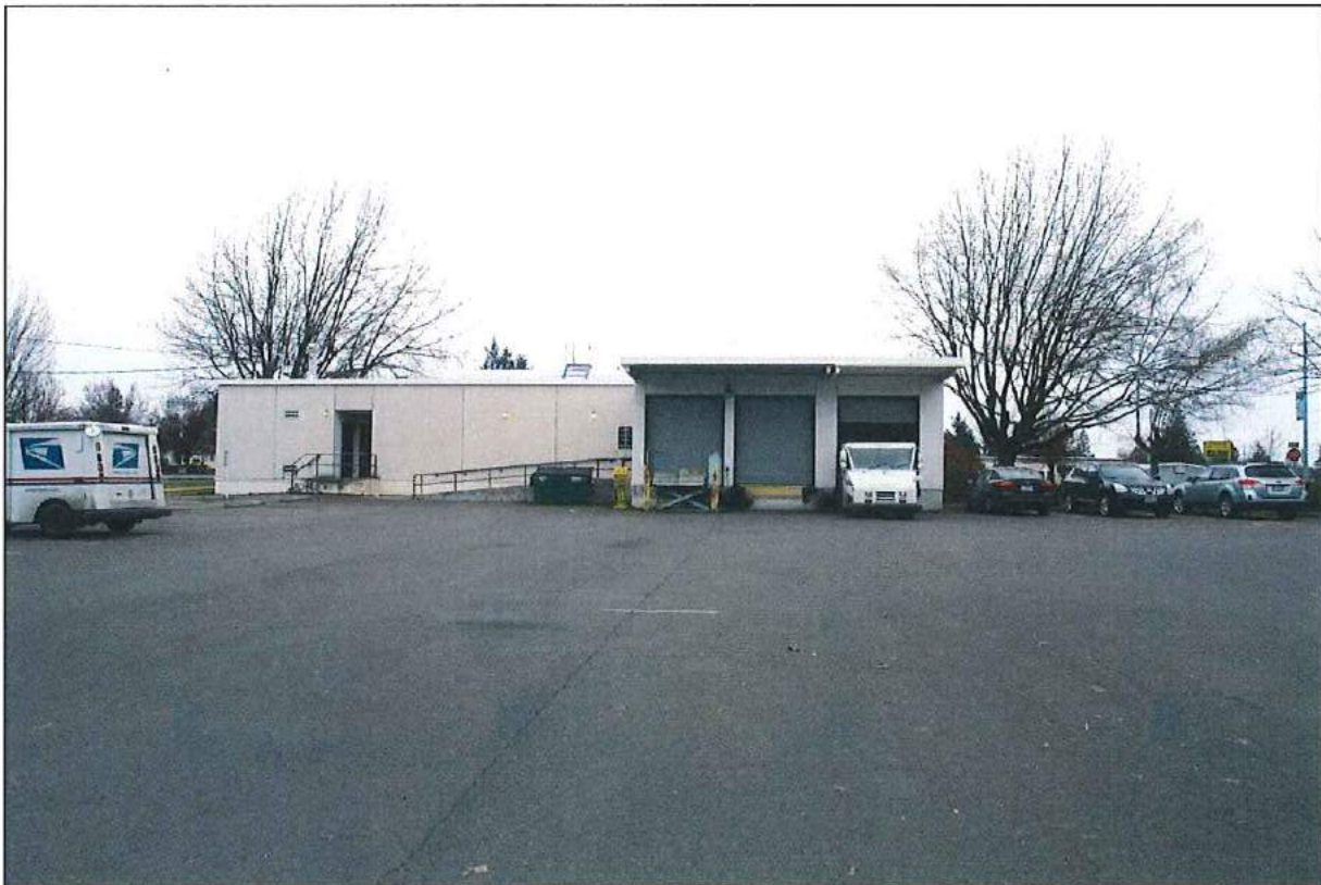
Photo 4 of 11: Exterior View, West Façade (rear), loading dock addition to the south, camera looking east
