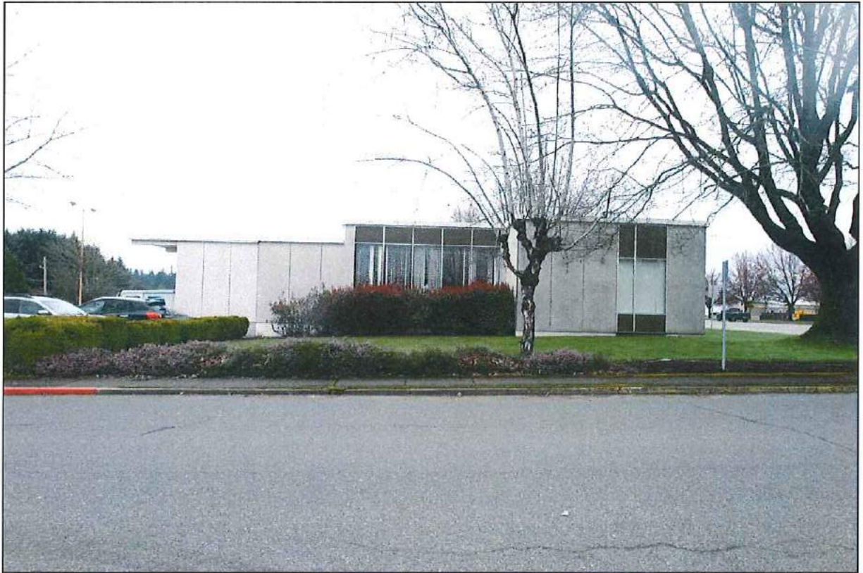
Photo 5 of 11: Exterior View, South Façade, loading dock addition to the west, camera looking north
