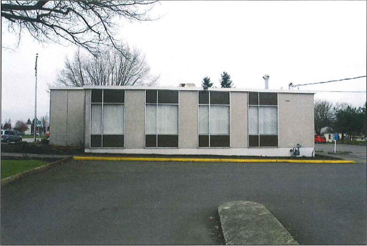
Photo 3 of 11: Exterior View, North Façade, camera looking south
